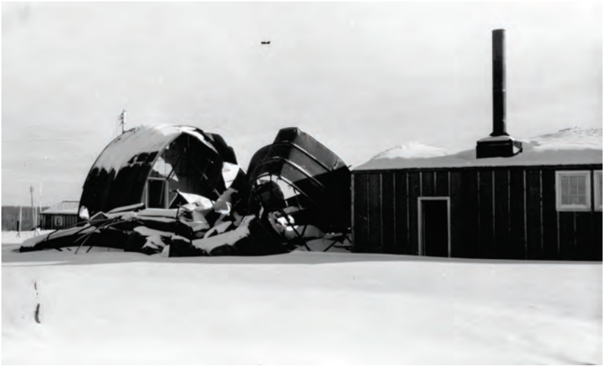
Figure 5-7: Effect of snow on Nissen Hut at Fort Nelson
