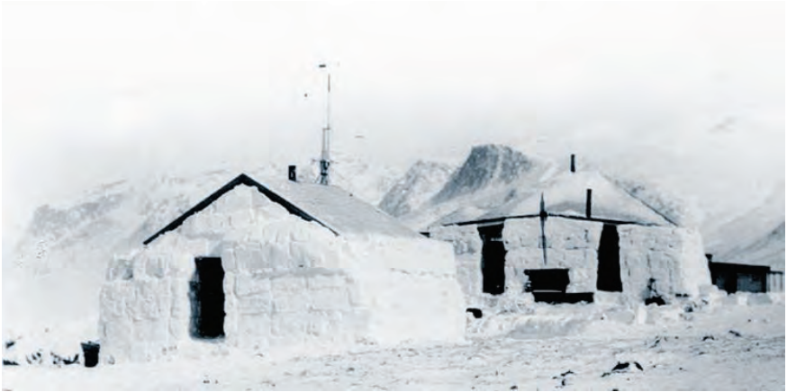
Figure 3-6: Ice blocks insulate huts in the north. Source: Hudson Strait Expedition/ Military Communications and Electronics Museum
